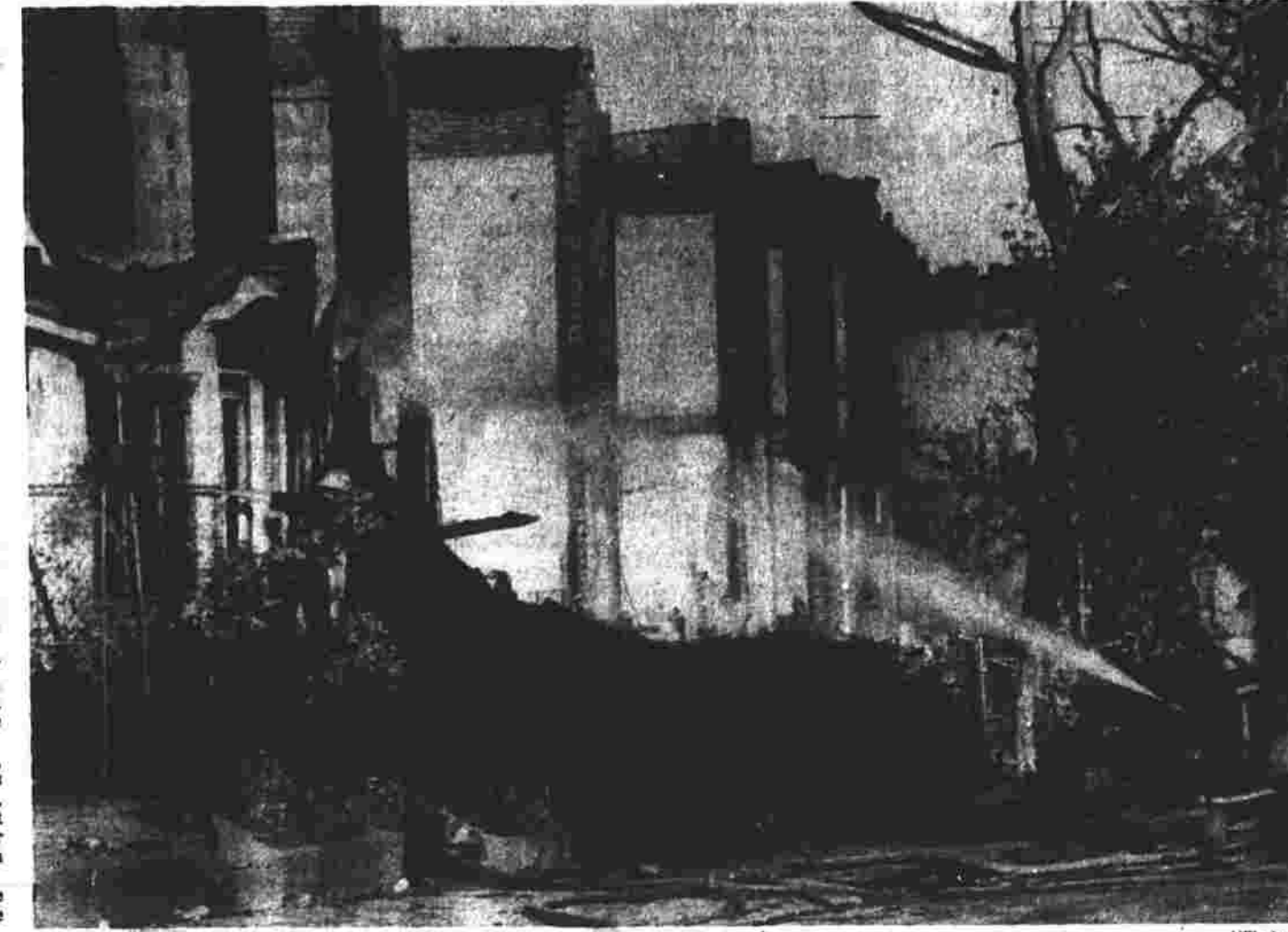
A Philadelphia fireman hoses down the remains of homes on Pine Street near the site of a shootout and fire that resulted from a confrontation between police and a radical back-to-nature group, MOVE, Monday. The fire was finally put out early this morning.
